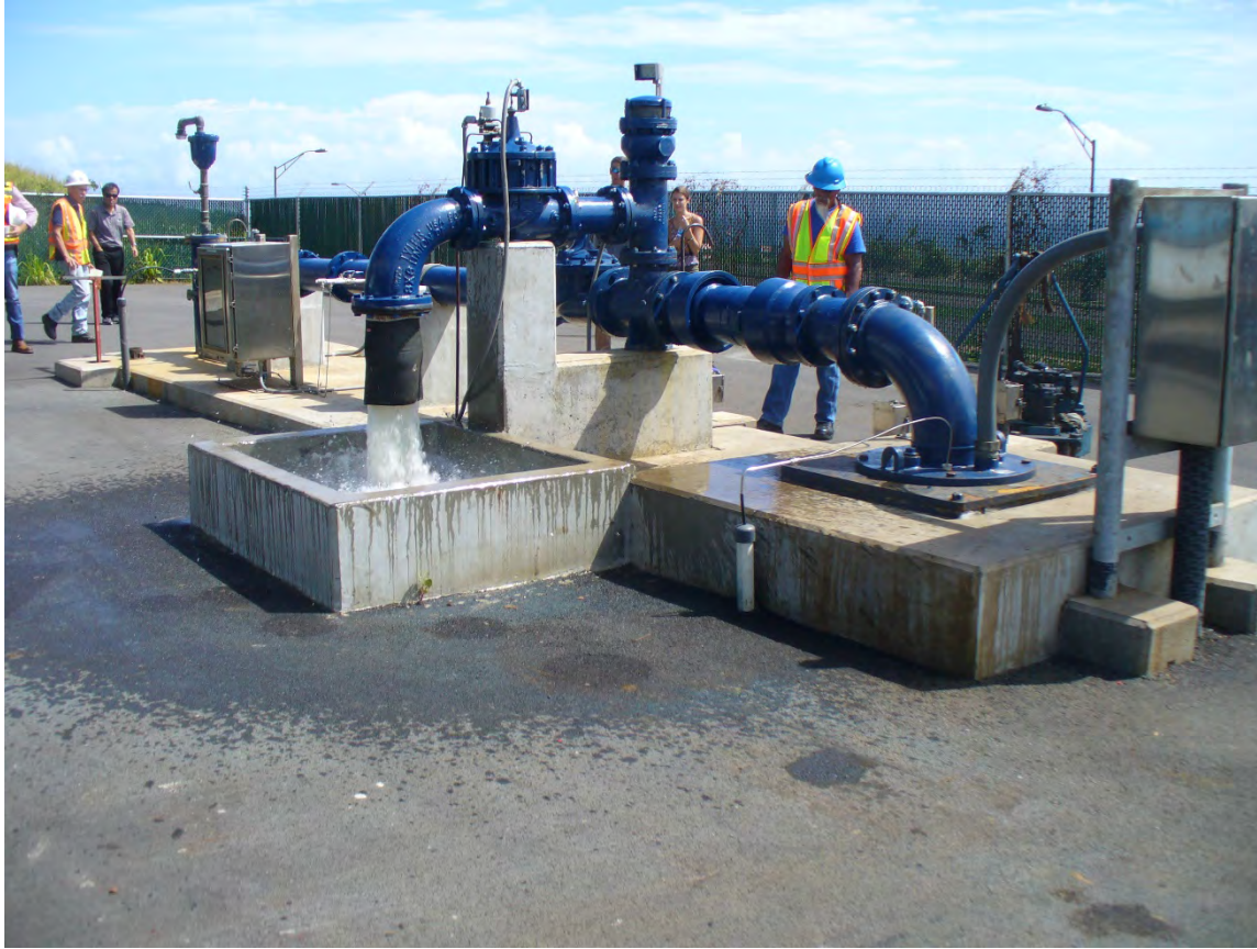
Start up and testing of Wailuku Well #2
